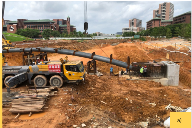
Figure 2. Key construction procedures: (a) installation of FCS DSTM arches, with CFST members connected to the arches; (b) casting of concrete into the FCS DSTM arch ribs with the steel and GFRP tubes as stay-in-place formwork; (c) installation of bridge deck system and UHPC cover.
