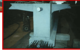
Figure 1. Beddington Trail Bridge.
