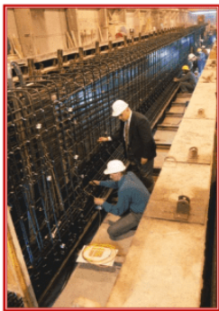
Instrumentation of the girder before casting
